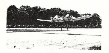
props. With the loss of air speed with one engine out the good engine could not develop its rated power. This is the reason ERCO recommended controllable pitch props.
